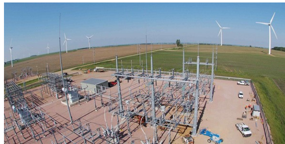
Xcel Energy upgrade project | Burns & McDonnell
